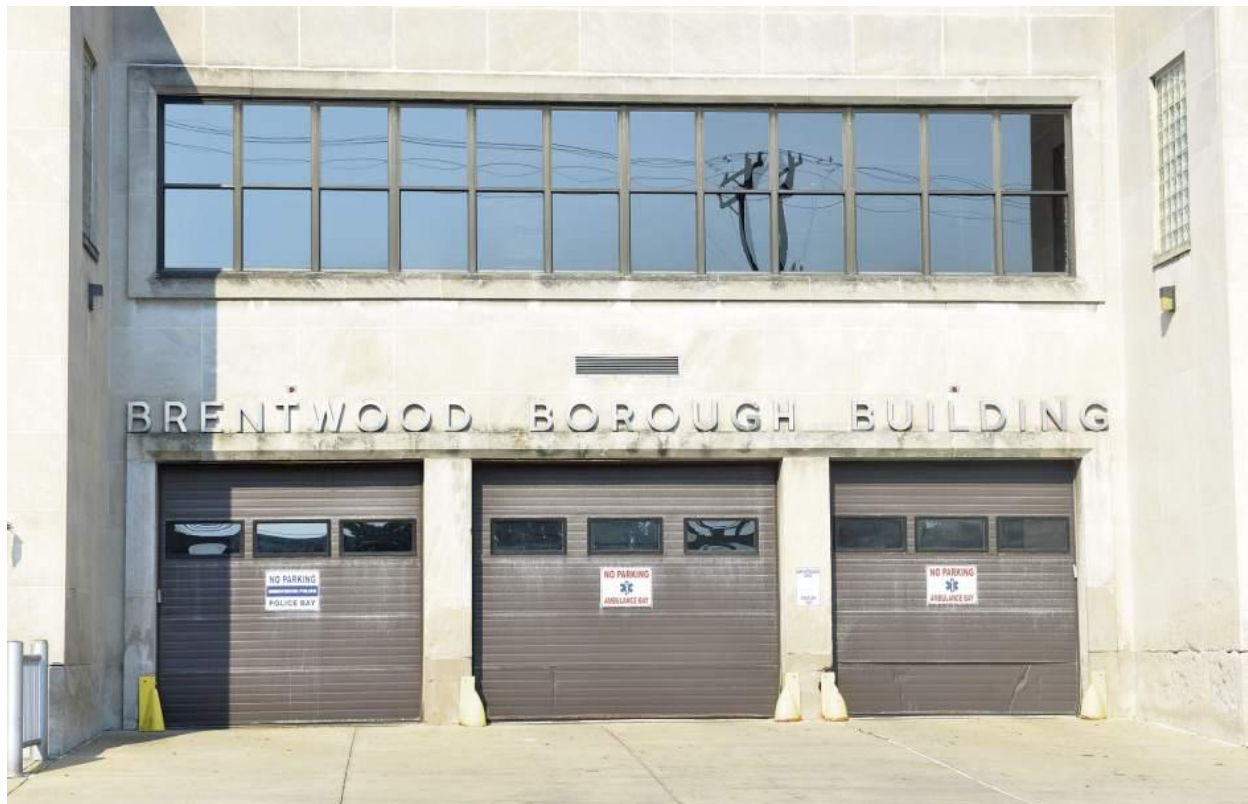
Brentwood Borough municipal building photographed Wednesday, July 19, 2017.
